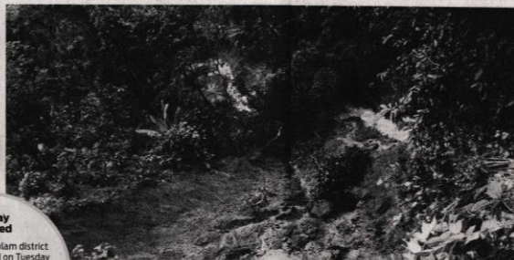
The landslide which occurred at Wagamon in Idukki on Monday | EXPRESS
