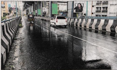
TALE OF CONTRAST: (LEFT) The Edappally flyover built by DMRC is intact, while the Palarivattom flyover constructed by RBDCCK is full of potholes. Both the flyovers were built using "high quality" bitumen macadam and dense bitumen macadam in 2016
