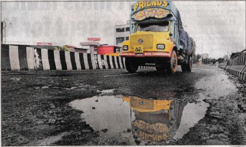
TALE OF CONTRAST: (LEFT) The Edappally flyover built by DMRC is intact, while the Palarivattom flyover constructed by RBDCCK is full of potholes. Both the flyovers were built using "high quality" bitumen macadam and dense bitumen macadam in 2016
