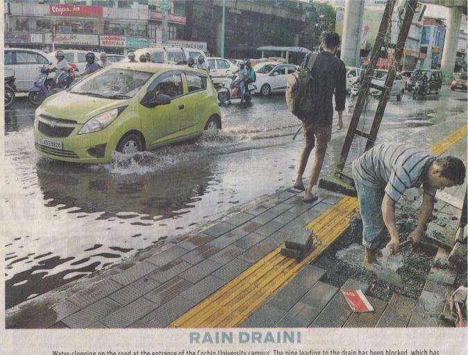
Water-clogging on the road at the entrance of the Cochin University campus. The pipe leading to the drain has been blocked, which has prompted workers to remove the newly laid tiles on the footpath to check the blockage | A SANESH
