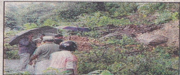
Landslip in Nadukani Ghat road
