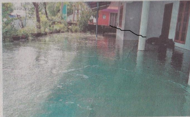
Floodwater that entered the premises of a house at Chellanam. ■SPECIAL ARRANGEMENT
