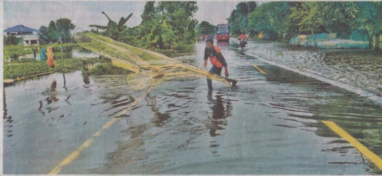
The Alappuzha-Changanassery road turned into a river, bringing traffic to a halt on Monday.
