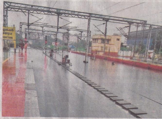
The flooded Ernakulam Junction railway station on Sunday.
